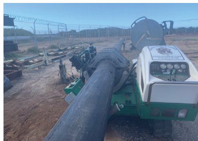
HDPE Fusion Equipment and Training
